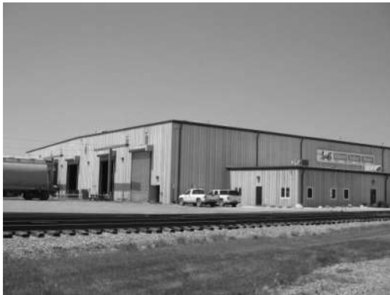
Midwest Railcar Repair in Corson promises energetic train enthusiasts a comprehensive, hour long walking tour of the 650 car capacity shop
