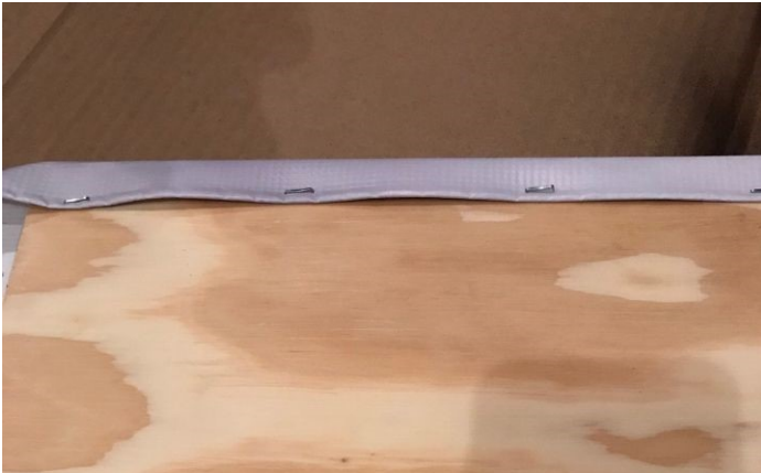
Photo 6: After the glue dried, staples were used to hold the vinyl to the back of the plywood.
