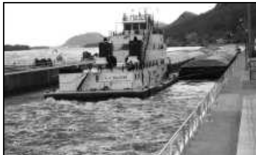
L. J. Sullivan at Lock & Dam No. 7
